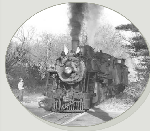
Locomotive at Monument Street, 1951
